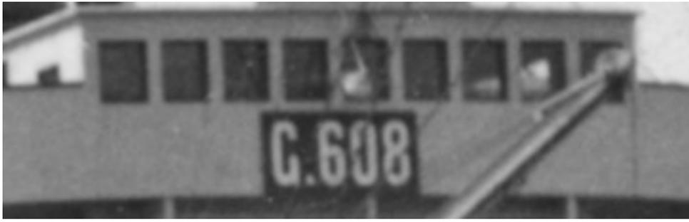
*Britannic's* bridge front as it looked early in 1916, which shows the number 'G.608'. Sometimes written without the full stop (or 'period' as they say in America), the number was displayed with one on the ship herself. The overhead lamp is positioned to illuminate the number at night. (Photo courtesy J & C McCutcheon collection/*The 'Olympic' Class Ships: Olympic, Titanic & Britannic* by Mark Chirnside.)
